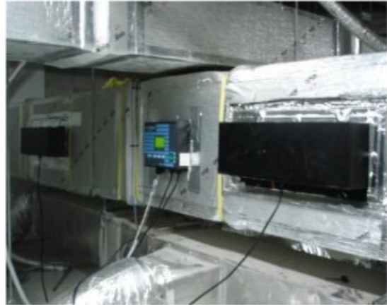
Installation Picture (Duct In Type for animal test labs)
